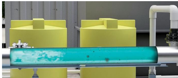
KAUST-developed anaerobic membrane bioreactor (AnMBR) technology
